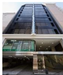
A-64 Alte Building Higobashi
