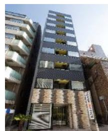
A-73 TENSUO OFFICE SHINBASHI 5
