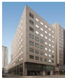
A-53 Sumitomo Mitsui Bank Koraibashi Building
