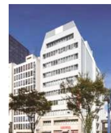
A-41 I-S Minamimorimachi Building
