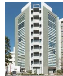
A-59 Yusen Higashi-Nihombashi Ekimae Building
