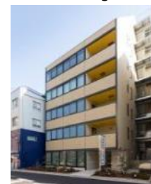
A-66 TENSJO OCHANOMIZU BUILDING
