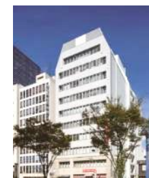
A-41 I-S Minamimorimachi Building
