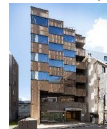
A-68 NRT Kandasudacho Building
