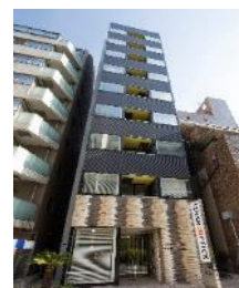
A-73 TENSJO OFFICE SHINBASHI 5
